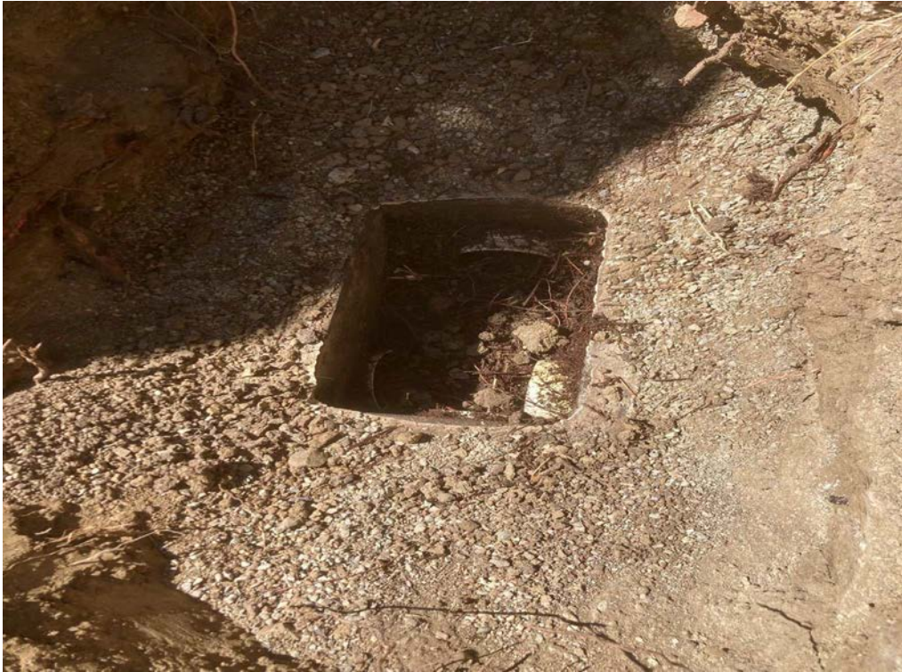
Photo 5: OWS 2 Distribution Box with Redwood Tree Roots Intrusion
