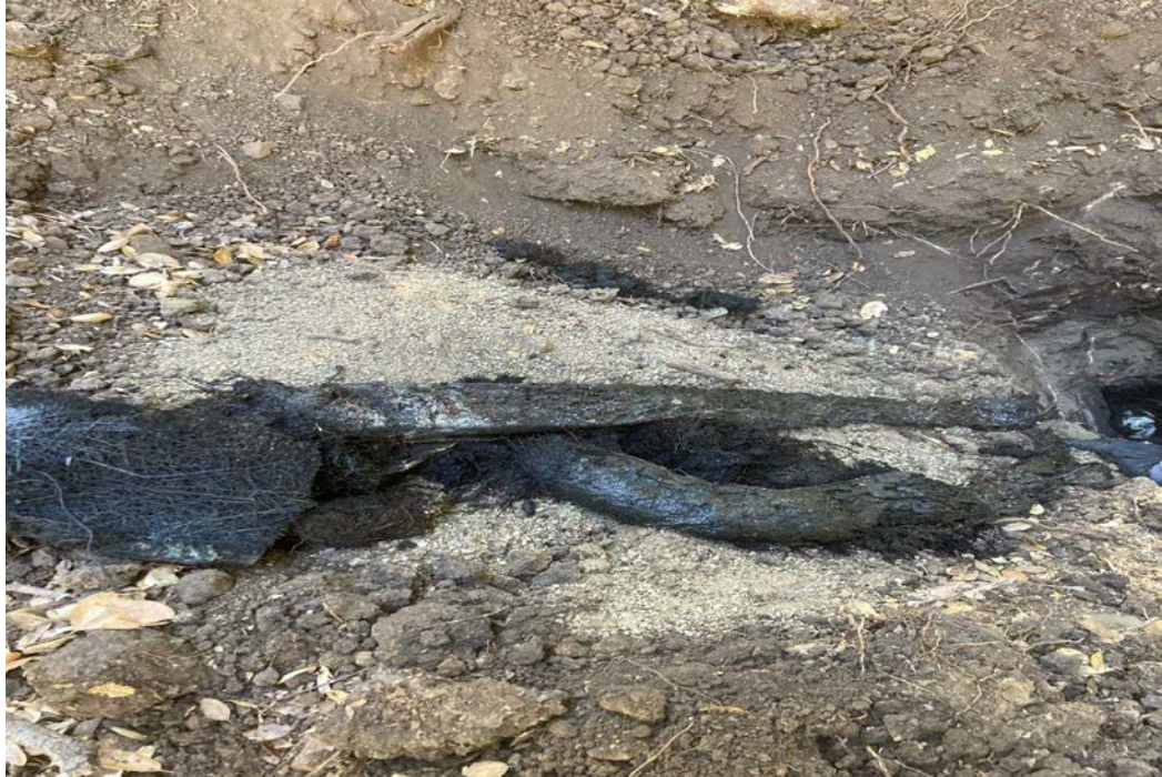
Photo 2: OWS 1 Roots Removed from Distribution Box and Distribution Laterals
