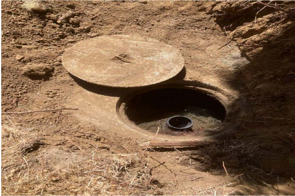
Photo 4: OWS 2 Septic Tank Second Compartment Outlet Sanitary Tee and Roots Intrusion
